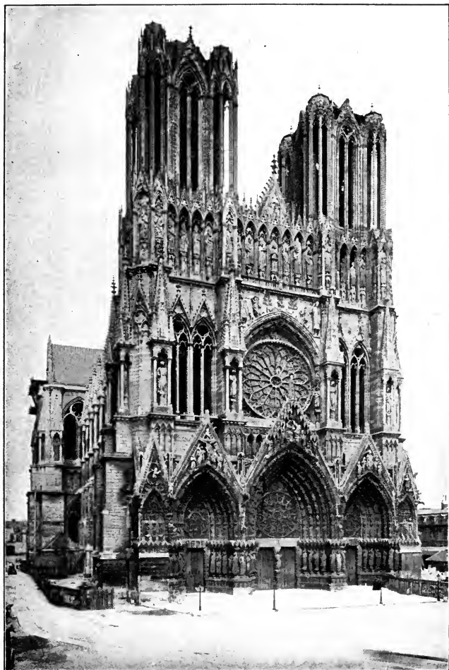
FAÇADE OF RHEIMS CATHEDRAL
